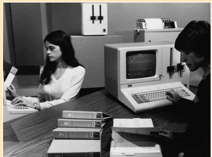
Figure 2. Datamaster, introduced in July 1981. Announced one month before the IBM PC, the System/23 Datamaster offered a viewing screen, keyboard, and diskette drives packaged in a single desktop console to support word processing and data processing in a machine that gave small businesses the big benefits of information processing.
