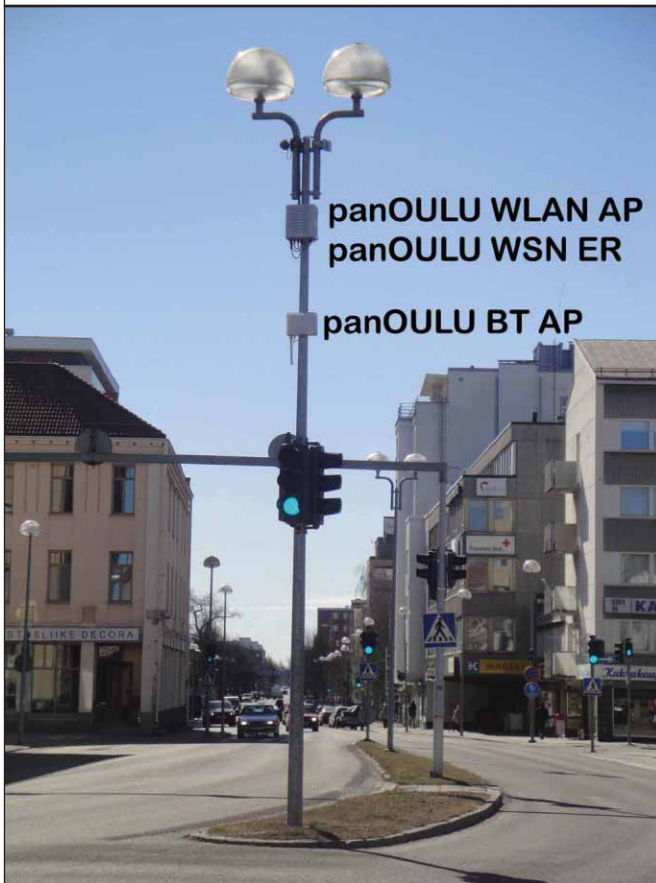
Figure 2. A panOULU wireless LAN access point (WLAN AP), wireless sensor network edge router (WSN ER), and Bluetooth access point (BT AP).
